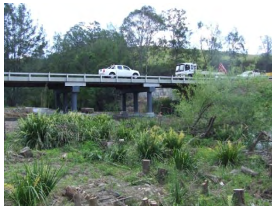
Figure 4: Leslie's Bridge replacement, Thunderbolts Way over the Manning River (Walcha-Gloucester)
