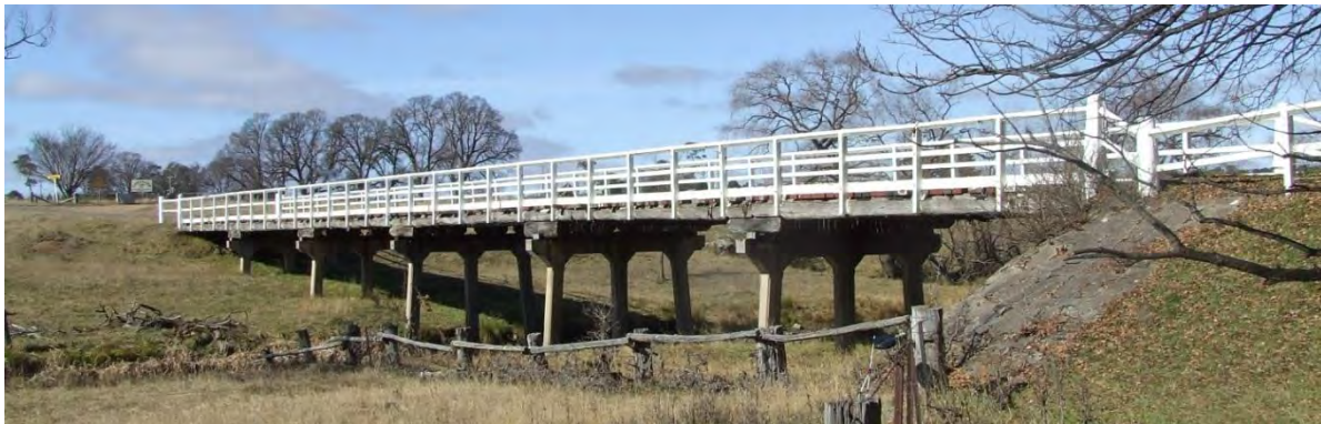
Figure 3: Munsie's Bridge over Salisbury Waters, east of Uralla
