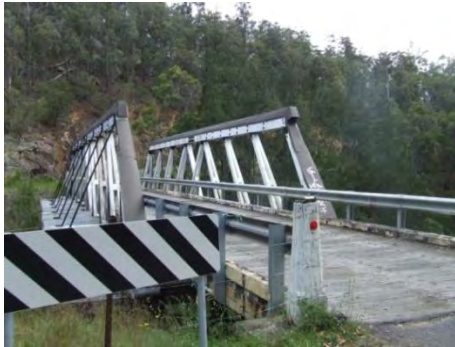
Figure 1: Bridge over Styx River
