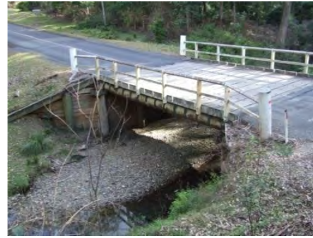
Figure 2: Horton's Creek Bridge, Armidale-Grafton Road
