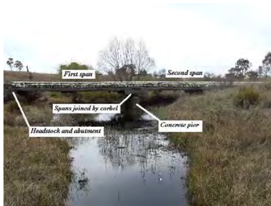
Photo 3: Multiple spans corbelled together, Uralla NSW
