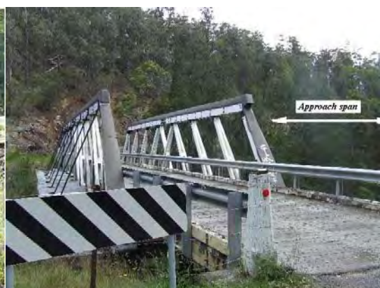
Photo 2: Example approach span, Styx River, Armidale-Kempsey Road, NSW
