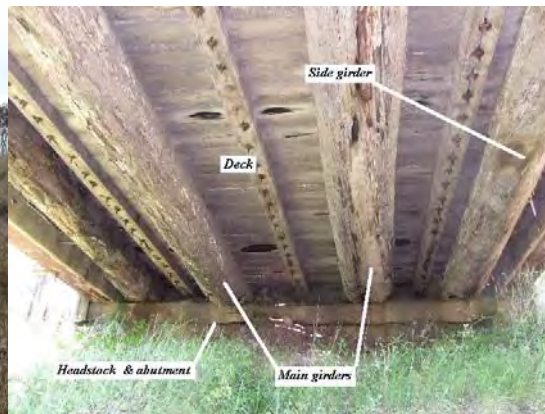
Photo 4: Underside of Styx river bridge approach section
