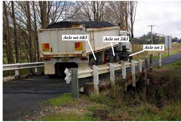
Photo 7: Stationary truck on bridge
